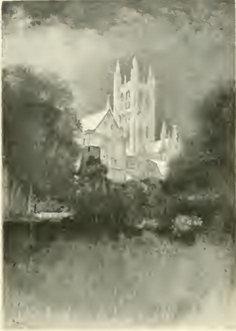
THE CENTRAL TOWER, FROM THE NORTHEAST.
